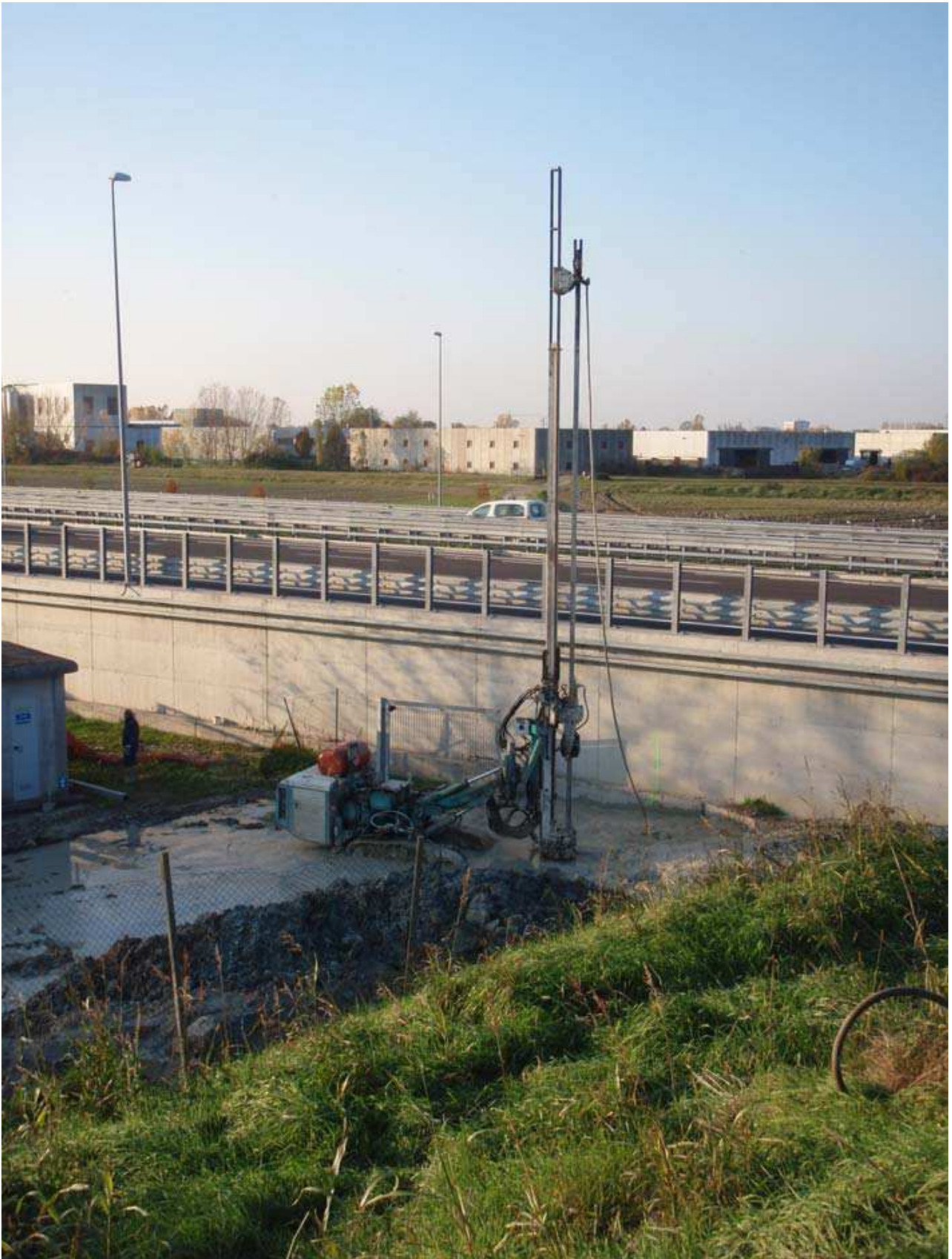
Lato Nord – Jet Grouting
